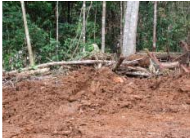
Figure 7. Soil and debris was often pushed into the forest.
