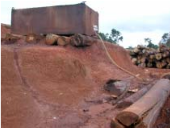
Figure 20. Diesel leaks are common at log camps. There was never any bunding or leak protection installed.
