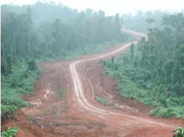
Figure 4. Road widths were often excessive.
