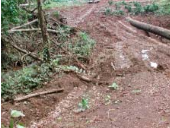
Figure 8. No water bars across steep skid tracks often led to severe erosion.
